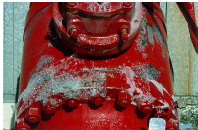
Figure 2: a soaping check for leaks
