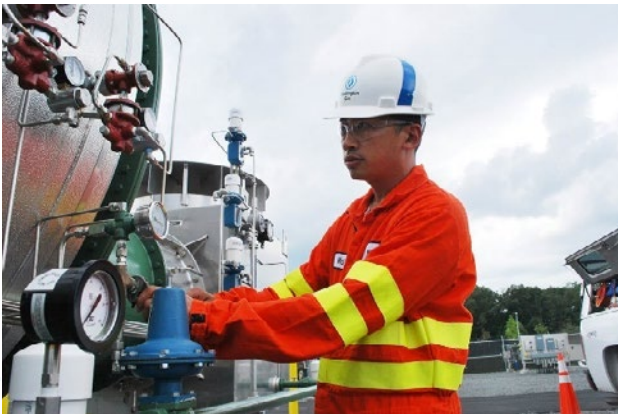
Figure 1 1 : Initial repairs being made
