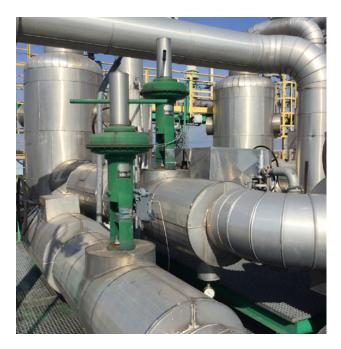
**Results:** The LTS technique only applies in plants where there is a significant difference in pressure between storage wells and the pipeline (for example, a 120-bar well and 20-bar pipeline). Where reasonably possible, Snam uses a refrigeration system with propane, or a lowtemperature separator process, instead of glycol dehydrators. Methane emission savings, compared to the use of glycol dehydrators, are estimated to be roughly 10.000 sm3 per year per storage site.
